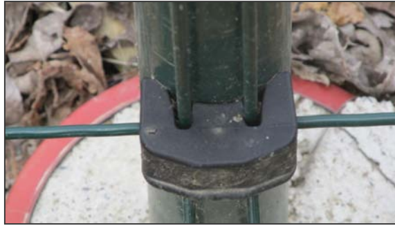
The fence must not move in the slots
