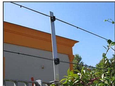
Example of L-shaped bracket with metal rope (diameter: 4mm)
