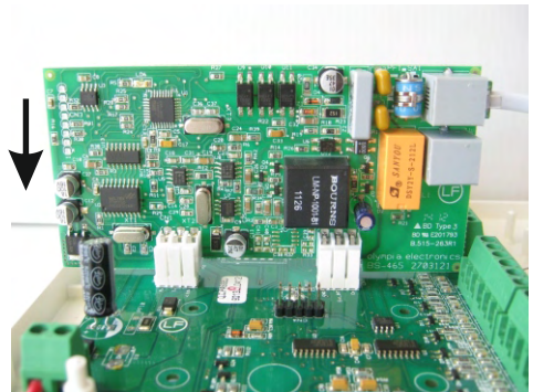
Figure 2 : Installing a BS-465 on the BS-468 panel
